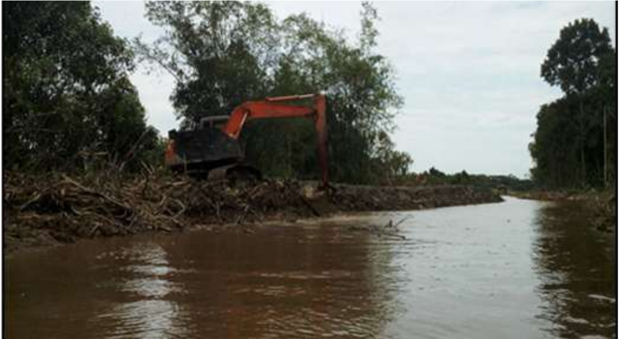
Figure 4: Clearing of river using the excavator to maintain water table
